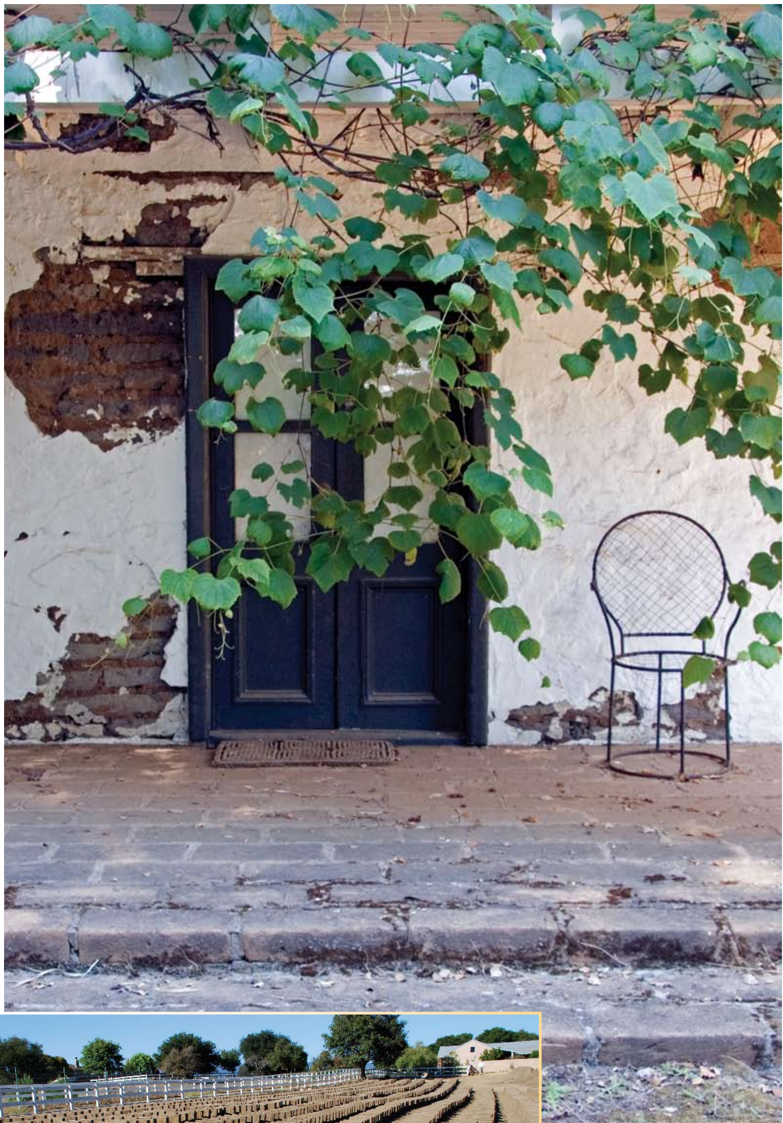
▲ Castro Adobe showing earthquake damage. Photo by John Goldberg ◀ Thousands of bricks were hand made by Friends volunteers. Photo by Jessica Kusz
