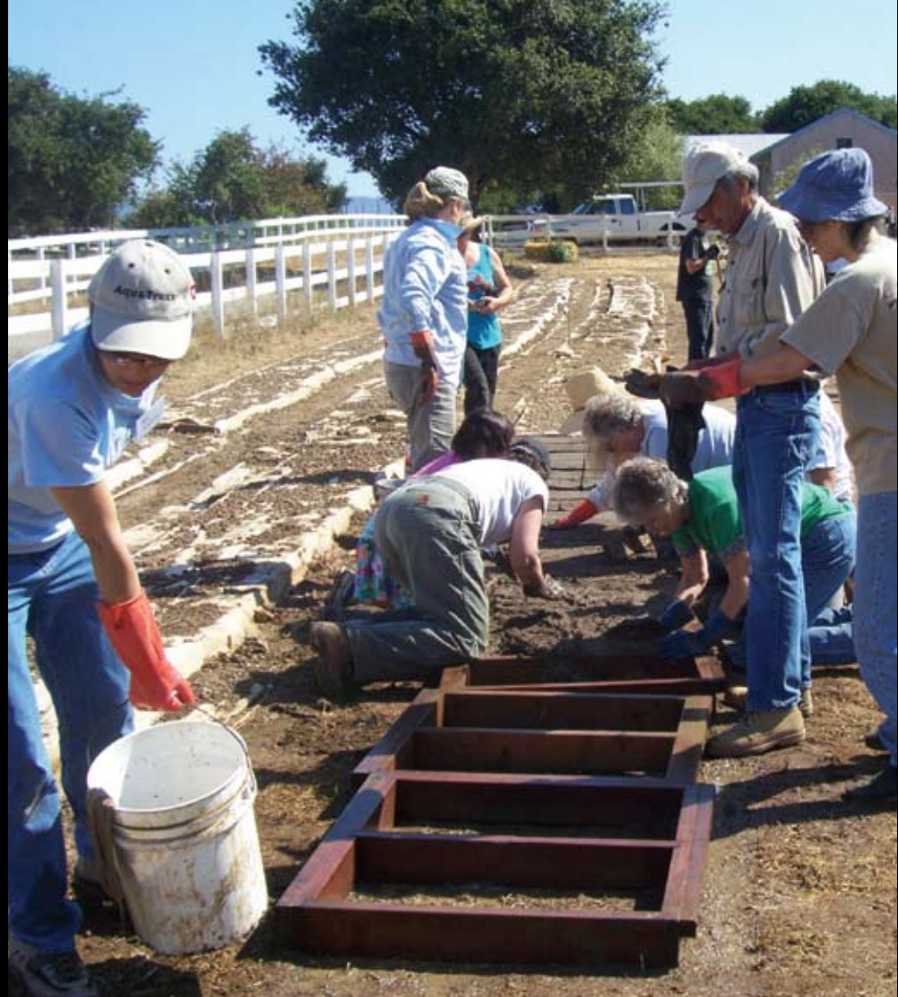
▲ Volunteers worked hard making adobe bricks using traditional methods guided by Tim Aguilar (in baseball hat). ▲ Bricks curing. Half of the bricks are standing while the others remain under paper & watered to slow drying process. All feature photos by Jessica Kusz, except where noted. ▲ The Castro Adobe prior to renovation. Photo by Cathy Rose
