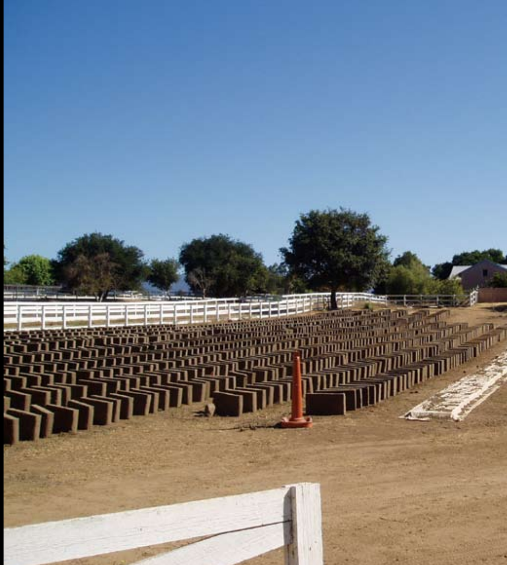
▲ Volunteers worked hard making adobe bricks using traditional methods guided by Tim Aguilar (in baseball hat). ▲ Bricks curing. Half of the bricks are standing while the others remain under paper & watered to slow drying process. All feature photos by Jessica Kusz, except where noted. ▲ The Castro Adobe prior to renovation. Photo by Cathy Rose
