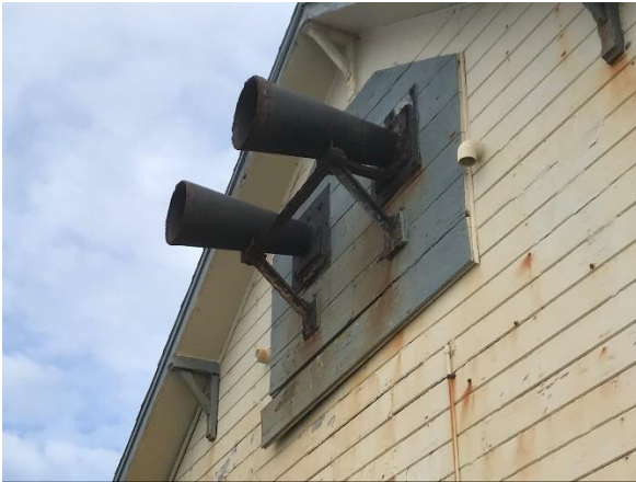
Before and after close-ups of exterior fog horns
